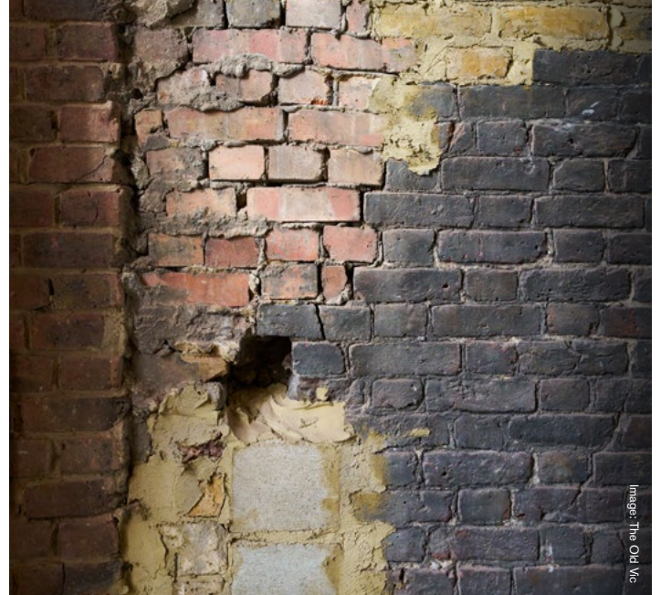
Exposed brickwork in the Clore Learning Centre
