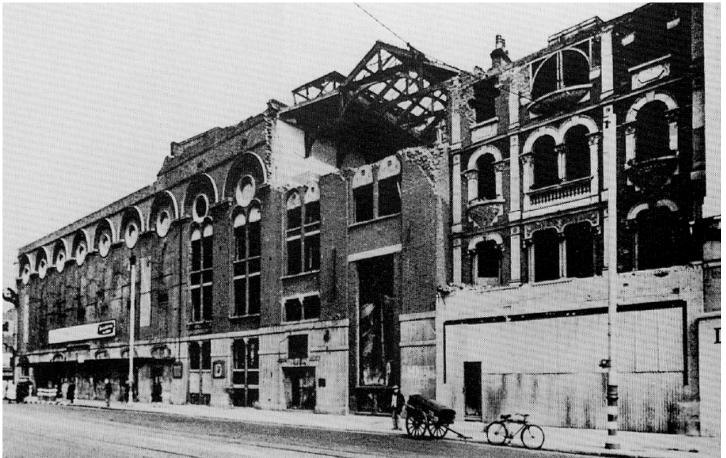
Bomb damage to 131 Waterloo Road, c.1941
