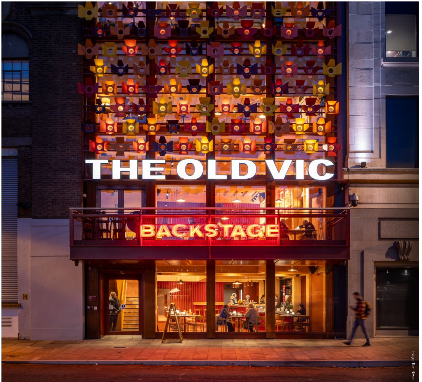
LED lights cast a warm glow across the Backstage façade at night
